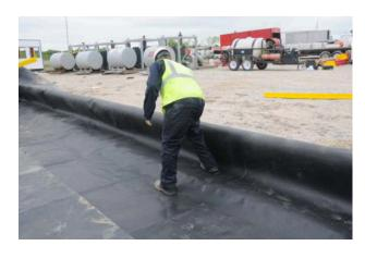
7. Walk around the containment area so that the liner lays close to the Containment Walls.
