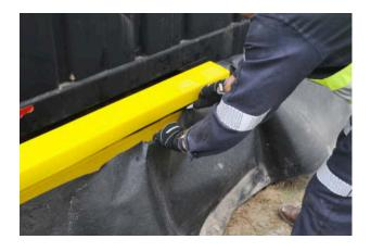
11. OPTIONAL: If desired, any excess liner material can be trimmed using a sharp utility knife.
