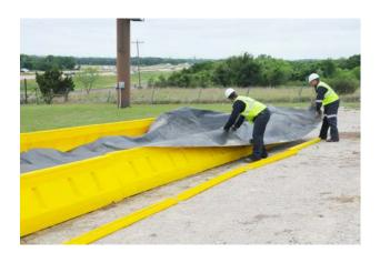
6. Once the pieces of the three walls have been connected, unfold the liner and lay it over the walls of the system.
