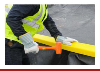
Place clips (two per wall / one per corner) over liner to secure it in place.
