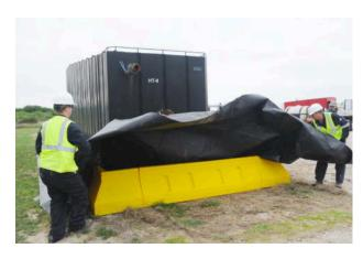
10. Once truck and/or any other equipment that will not be contained is removed, replace any walls/corners that were removed in step 4. Install clips.
