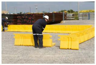
3. Set up walls and corners in area requiring spill containment.
