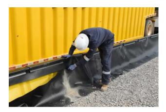
12. OPTIONAL: If desired, any excess liner material can be trimmed using a sharp utility knife.
