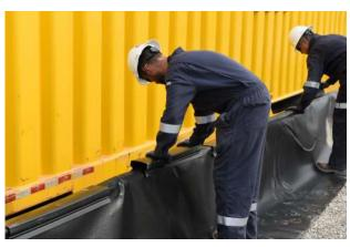
11. Place clips (two per wall / one per corner) over liner to secure it in place. (NOTE: The clips are designed to fit snugly and may require a fair amount of force to install. A rubber mallet can be helpful).
