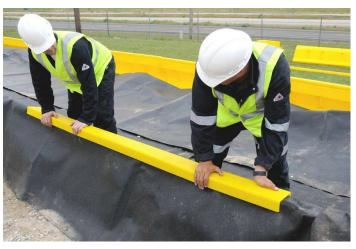
The 30 MIL polyethylene textured liner is held on the walls with 8-foot long clips. These clips snap over the liner and the straight section walls.
